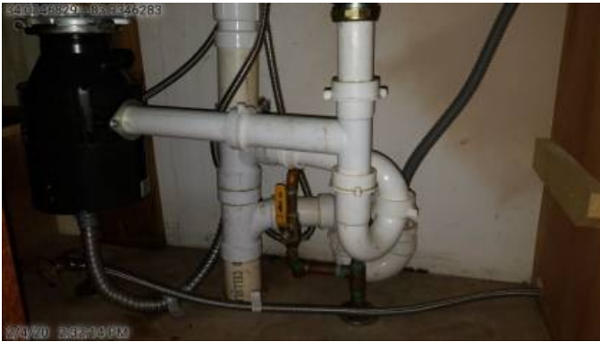
9.4 Kitchen Sink Cabinet / Countertop:
